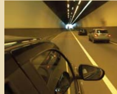
Rail and roadway tunnels
