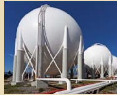
Chemical and flammable materials storage
